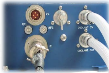
Figure 2-6 Laser Head Signal Connection
