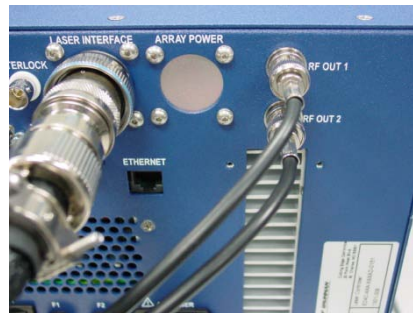
Figure 2-14 RF Signal Cables
